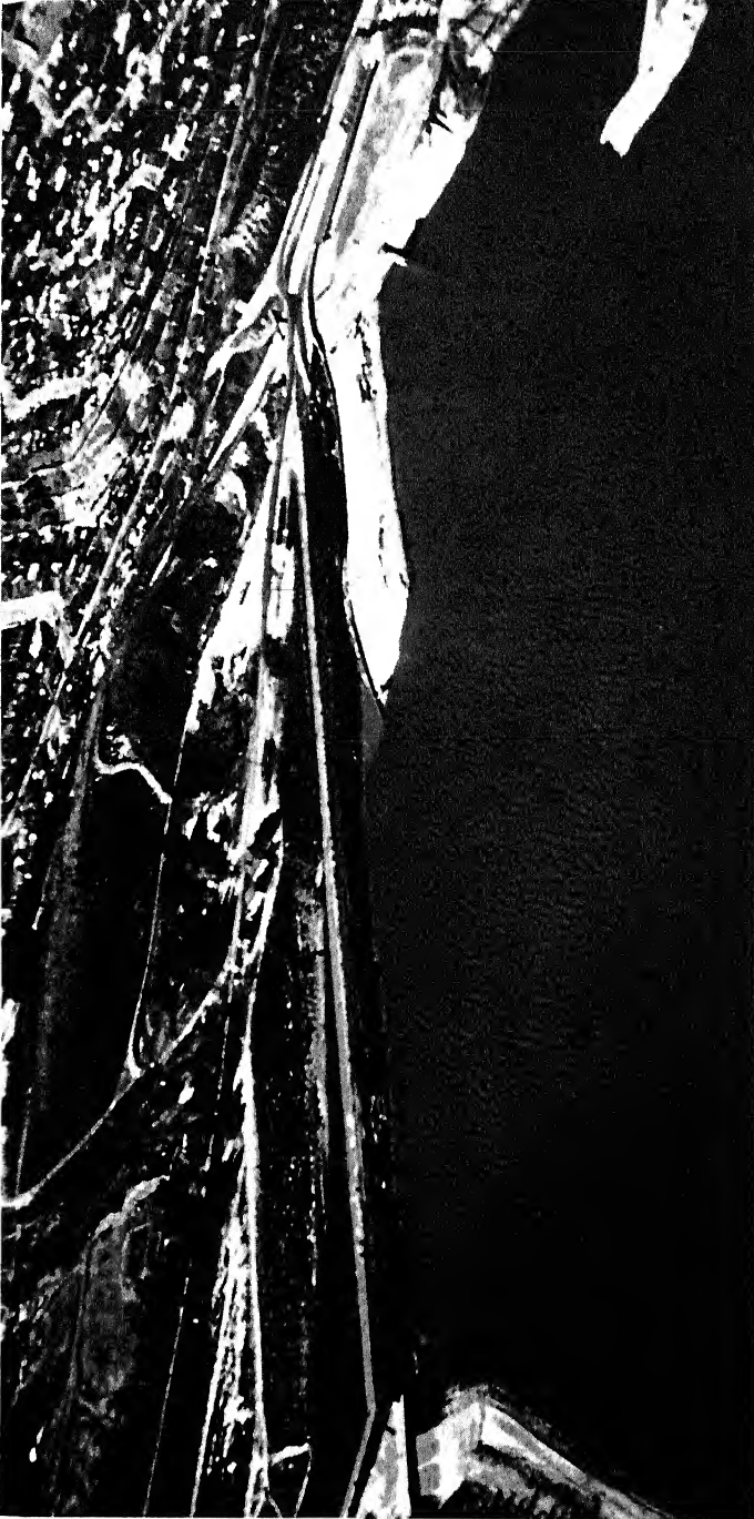
FIGURE 3.2 The lower Van Norman Dam, which was severely damaged by the February 9, 1971, San Fernando earthquake. 80,000 people living in the valley below the dam were evacuated because complete failure appeared imminent. (Photograph supplied by Bruce Bolt.)
