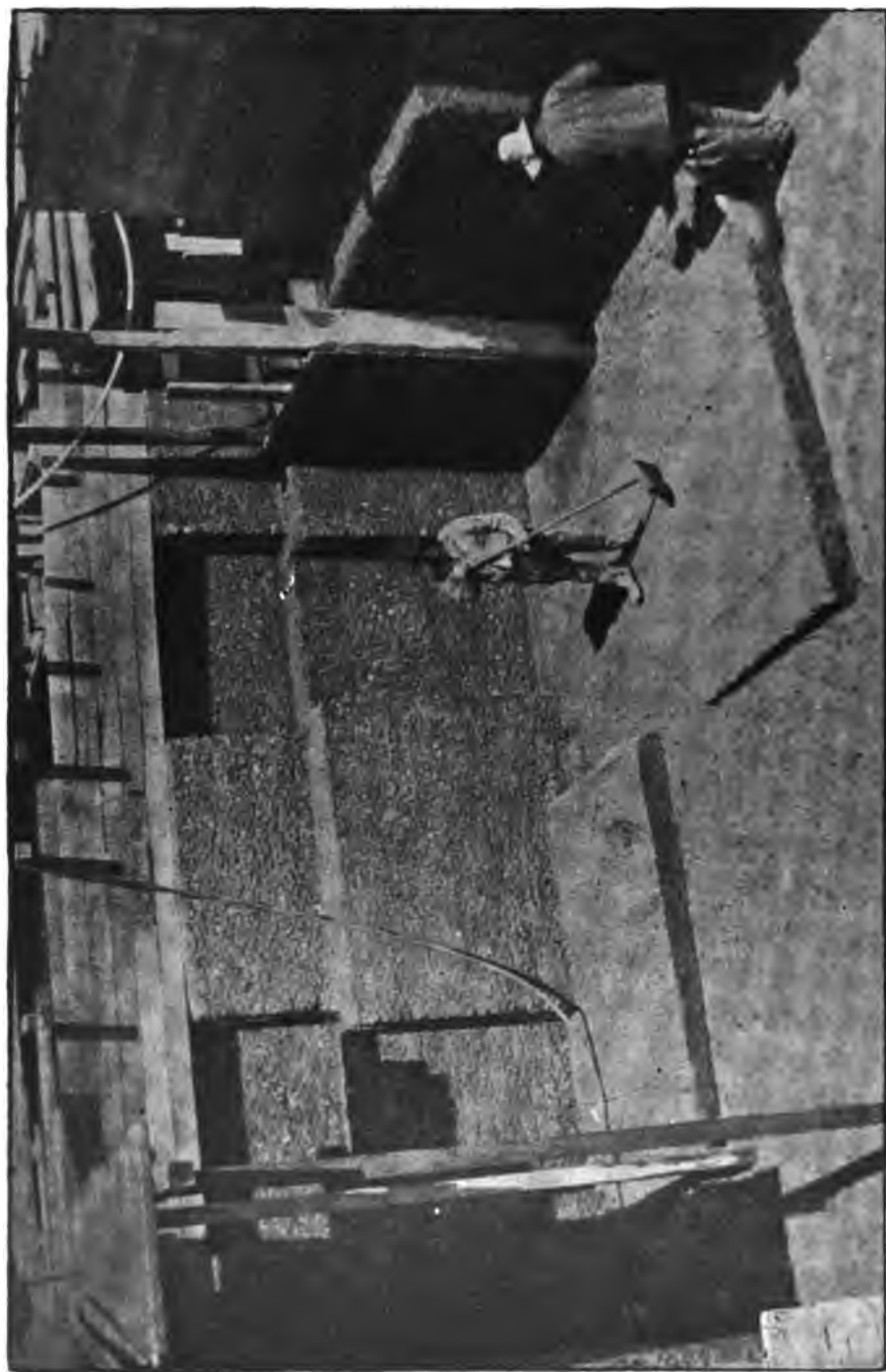
FIG 193.—ROUGHENING SURFACE OF CONCRETE BLOCKS TO RECEIVE FRESH CEMENT, AT SAN MATEO DAM.
