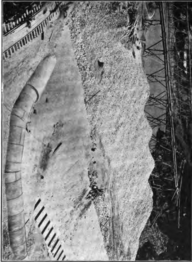
FIG. 126.—LOWER TOE OF NECAHA DAM, MEXICO, SHOWING CHARACTER OF HYDRAULIC-FILL MATERIAL. PIPE IN FOREGROUND IS 10 FEET IN DIAMETER, USED ONLY FOR FLOOD DISCHARGE DURING CONSTRUCTION.
