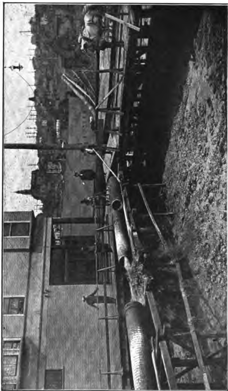
FIG. 354.—THE DELIVERY OF SLUICED MATERIAL TO FILL LOW GROUND IN THE REGRADING OF SEATTLE, WASH. 515
