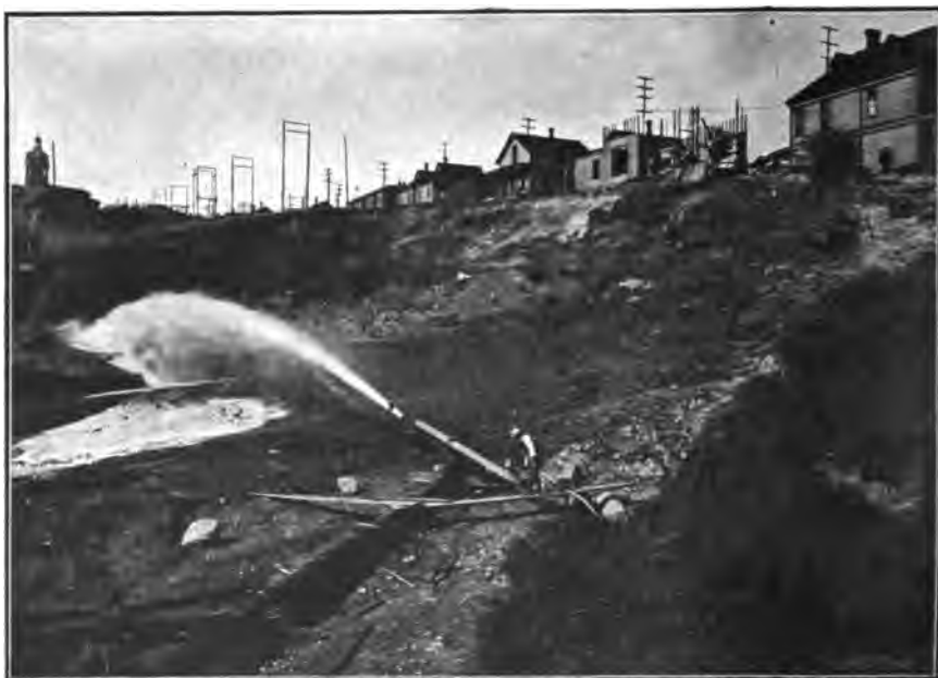
FIG. 352.—THE REGRADING OF JACKSON STREET, SEATTLE, LOOKING NORTH ON MAYNARD STREET. THE HOUSES ARE REMOVED JUST BEFORE THEY ARE UNDERMINED.
