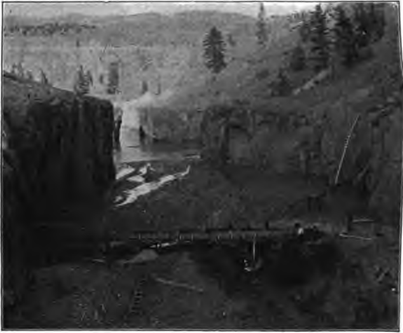
FIG. 104. —TERRACE DAM, COLORADO, LOOKING UP-STREAM. ILLUSTRATING GRADATION OF MATERIAL TOWARD THE CENTER OF THE DAM FROM THE POINT OF DEPOSIT AT THE SLOPES.
