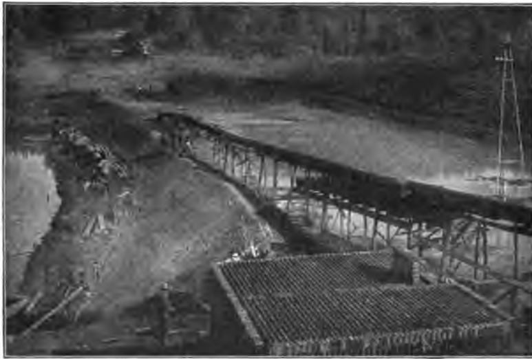
FIG. 86.—TOE LEVEE OF NORTH FACE, LAKE FRANCES DAM, AND INLET CRIB AT HEAD OF FIVE-FOOT OUTLET CULVERT.
