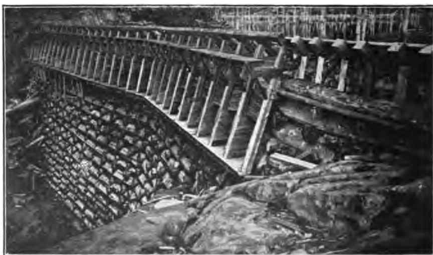
FIG. 340.—TIMBER CRIB SPILLWAY OF BOWMAN LAKE DAM. THIS STRUCTURE IS 52 FEET HIGH.
