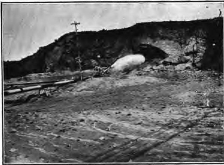
FIG. 110.—SANTO AMARO DAM, BRAZIL, SHOWING HYDRAULIC MONITOR AT WORK, DELIVERING 8 SECOND-FEET UNDER 85 POUNDS PRESSURE THROUGH 4-INCH NOZZLE.
