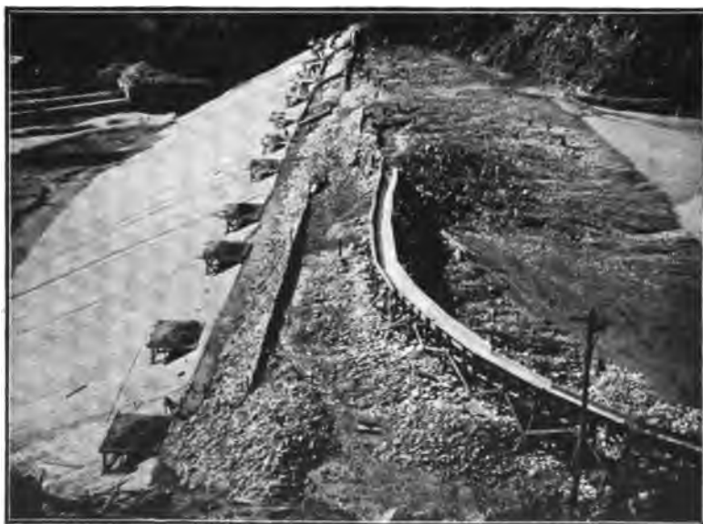
FIG. 121.—DOWN-STREAM SLOPE OF NECAXA DAM, SHOWING MASONRY PAVEMENT ON FACE AND CHARACTER OF SLUICED MATERIAL.
