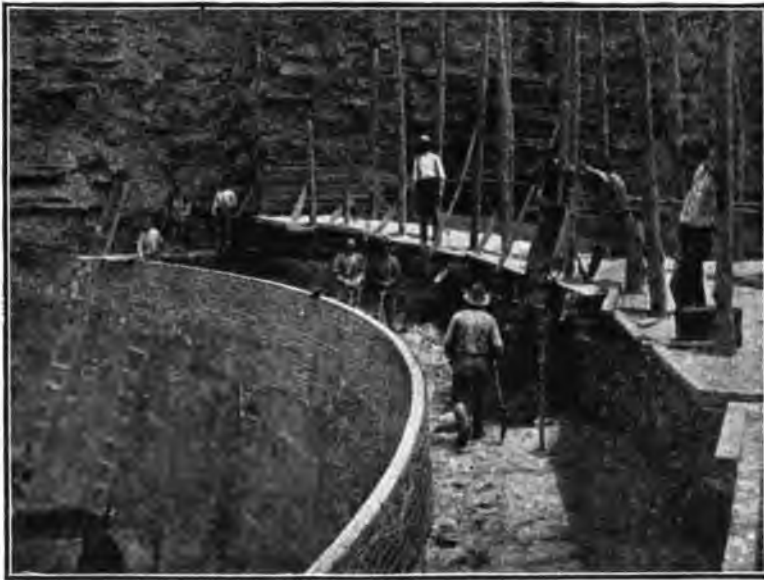
FIG. 222.—ITHACA DAM, NEW YORK, ILLUSTRATING CONCRETE CONSTRUCTION BETWEEN BRICK-FACING FORMS.
