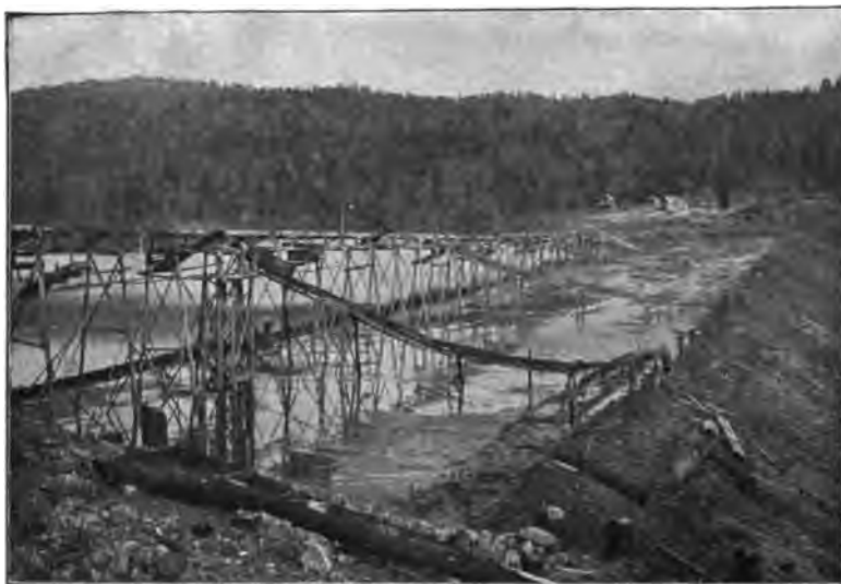
FIG. 92.—LAKE FRANCES, CAL., HYDRAULIC-FILL DAM BUILDING. SHOWING OUTER LEVEES MAINTAINED WITH BRUSH, DEFLECTING BOARDS FOR DISTRIBUTING SLUICINGS ALONG SLOPE, GENTLE SLOPES TOWARD CENTER OF DAM, AND GRADUAL MOVEMENT OF DRAINAGE TOWARD EXTREME END.
