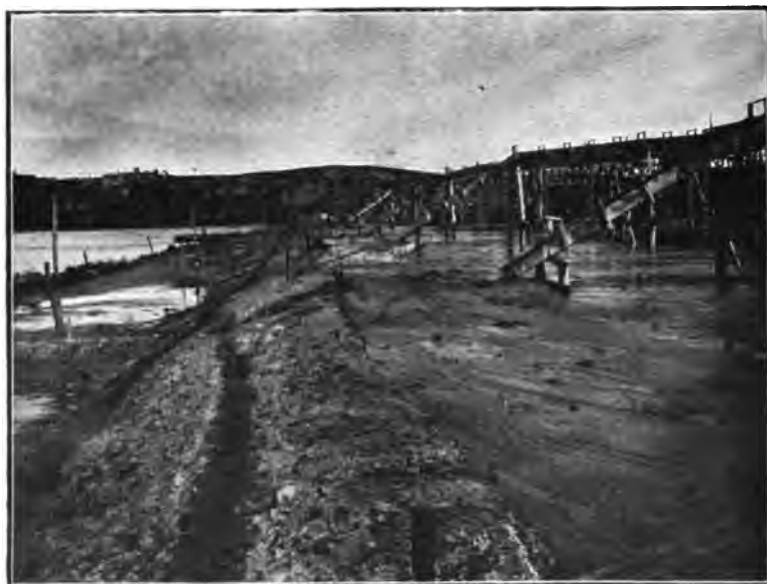
FIG. 111.—UPPER TOE FILLING ON THE SANTO AMARO HYDRAULIC-FILL DAM, BRAZIL, SHOWING LATERAL FLUMES.
