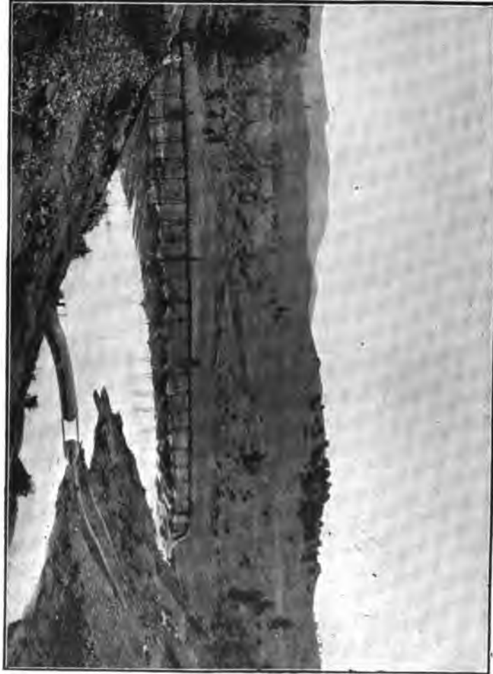
Fig. 102.—TERRACE DAM, COLO., SHOWING DEPOSIT OF STICED MATERIAL ON UP-STREAM TOE OF DAM. THE ABANDONED CORE-WALL, 70 FEET HIGH, SHOWS JUST OUT OF WATER.
