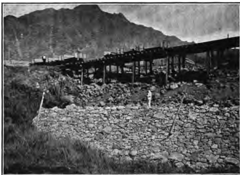
FIG. 100.—NUUANU DAM, HONOLULU, SHOWING TOE OF ROCK-FILL PORTION OF DAM.
