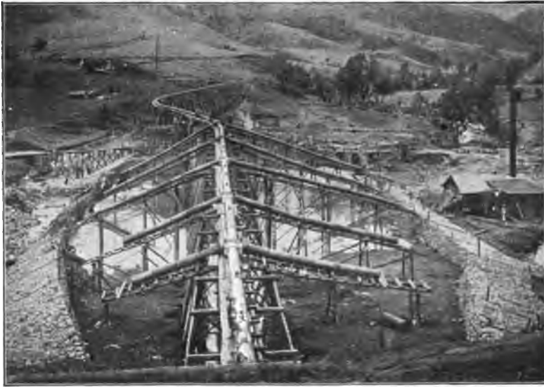
FIG. 132.—METHOD OF DISTRIBUTING SLUICED MATERIALS THROUGH PIPES, DAM No. 1, AT ACATLAN, TENANGO RIVER.
