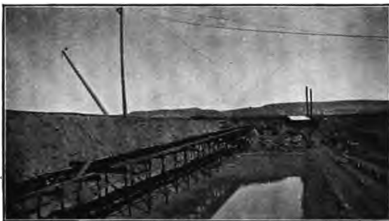
FIG. 59.—ZUÑI DAM, N. M., ILLUSTRATING METHOD OF DELIVERY OF SLUICED MATERIALS BY "V" FLUME, AGAINST FACE OF ROCK-FILL.
