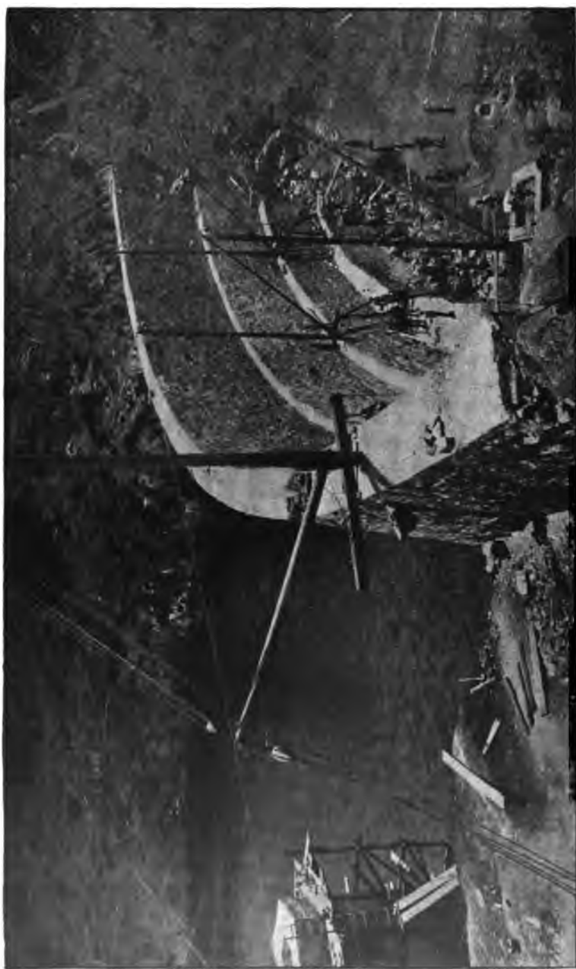
FIG. 150.—ORIGINAL SWEETWATER DAM AS COMPLETED TO THE SIXTY-FOOT CONTOUR.
