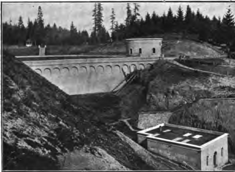
FIG. 212.—CONCRETE DAM, 60 FEET HIGH, AT RESERVOIR NO. 3, PORTLAND, ORE. POWER-HOUSE IN FOREGROUND.
