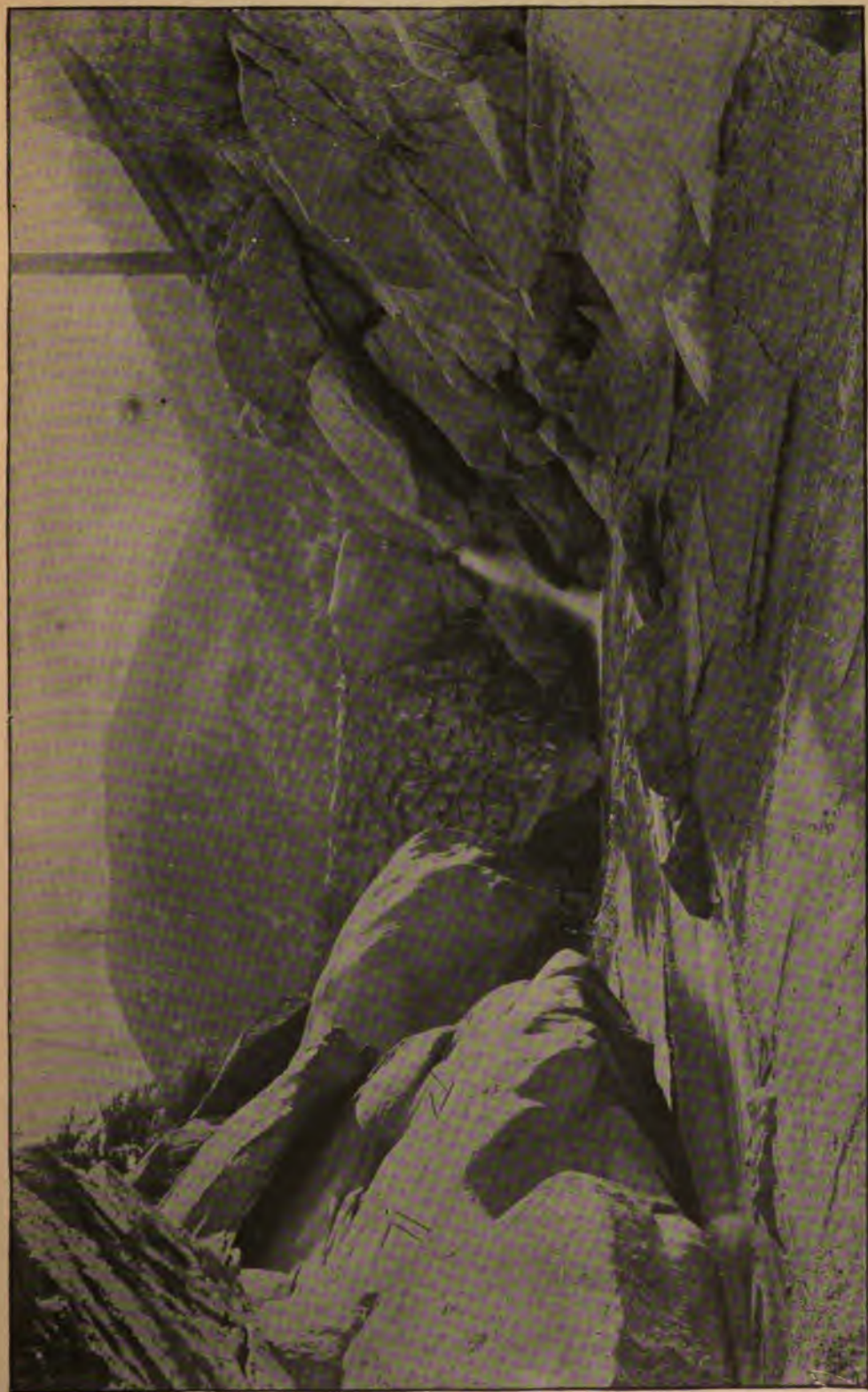
FIG. 20.—THE BARRETT DAM-SITE, SHOWING THE BEGINNING OF MASONRY FOUNDATIONS. The material on left bank above the rock here shown is disintegrated granite to such depth as to require change of plans from original design.
