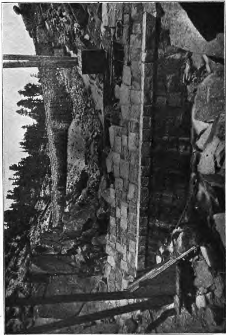
FIG. 176.—BASE OF NEW ROCK-FILL DAM, BELOW THE BEAR VALLEY DAM (SHOWN IN BACKGROUND).
