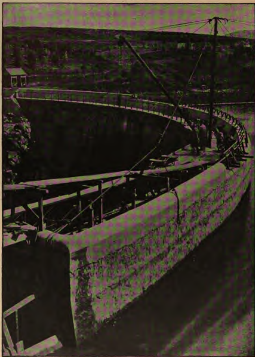
FIG. 159.—REPAIRING AND INCREASING THE HEIGHT OF THE PARAPET OF SWEET-WATER DAM.
