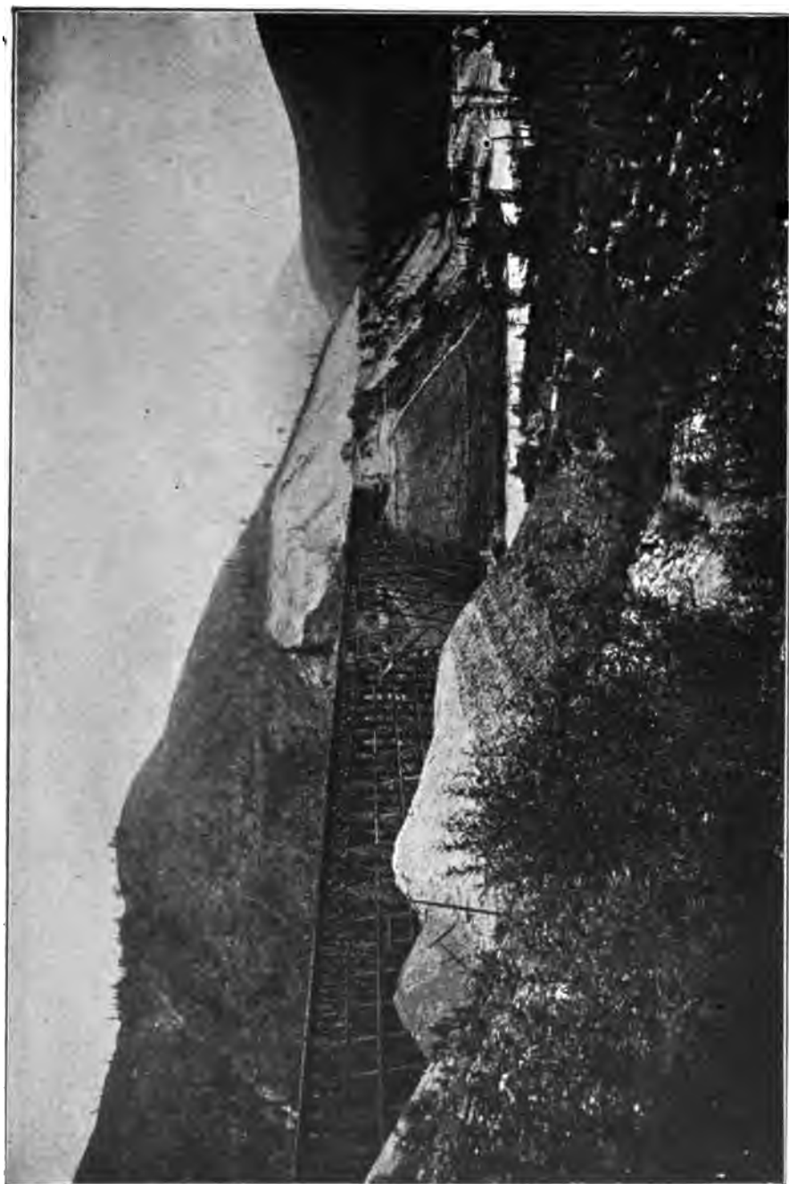
FIG. 141.—HYDRAULIC FILLS, PARTIALLY COMPLETED, AT MOUNTAIN CREEK, B. C., CANADIAN PACIFIC RAILWAY.
