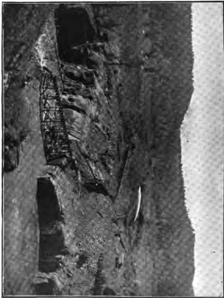
FIG. 107.—VIEW OF LOWER TOE FILLING, TERRACE DAM, COLORADO, SHOWING HYDRAULIC SLICING IN BACKGROUND.
