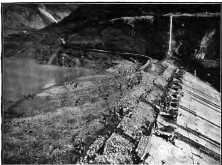
FIG. 120.—LOWER TOE OF NECAXA DAM, LOOKING NORTH, SHOWING DELIVERY OF ROCK AND CLAY BY FLUME.
