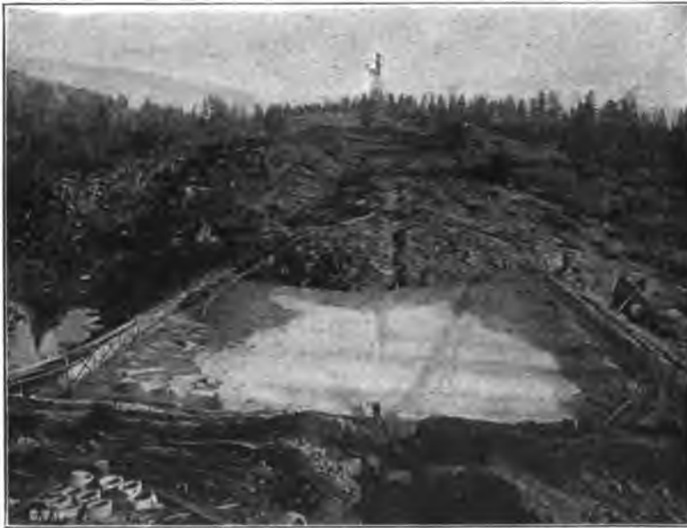
FIG. 80.—CRANE VALLEY DAM SHOWING DISCHARGE OF SLUICED EARTH AT END OF CONVEYING FLUME.
