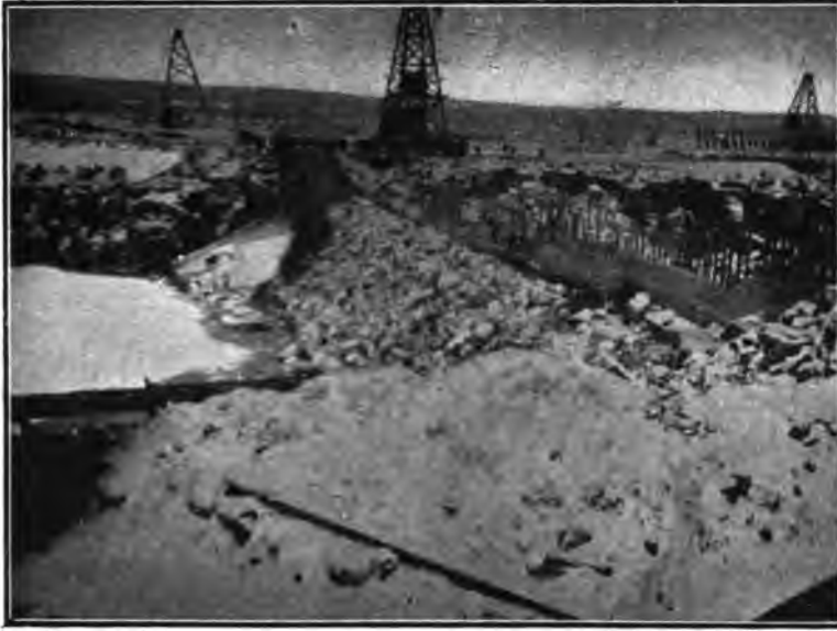
FIG. 51.—MILNER DAM, SNAKE RIVER, IDAHO. SHOWING ROCK-FILL WITH WOOD-CORE IN MAIN CHANNEL OF RIVER.
