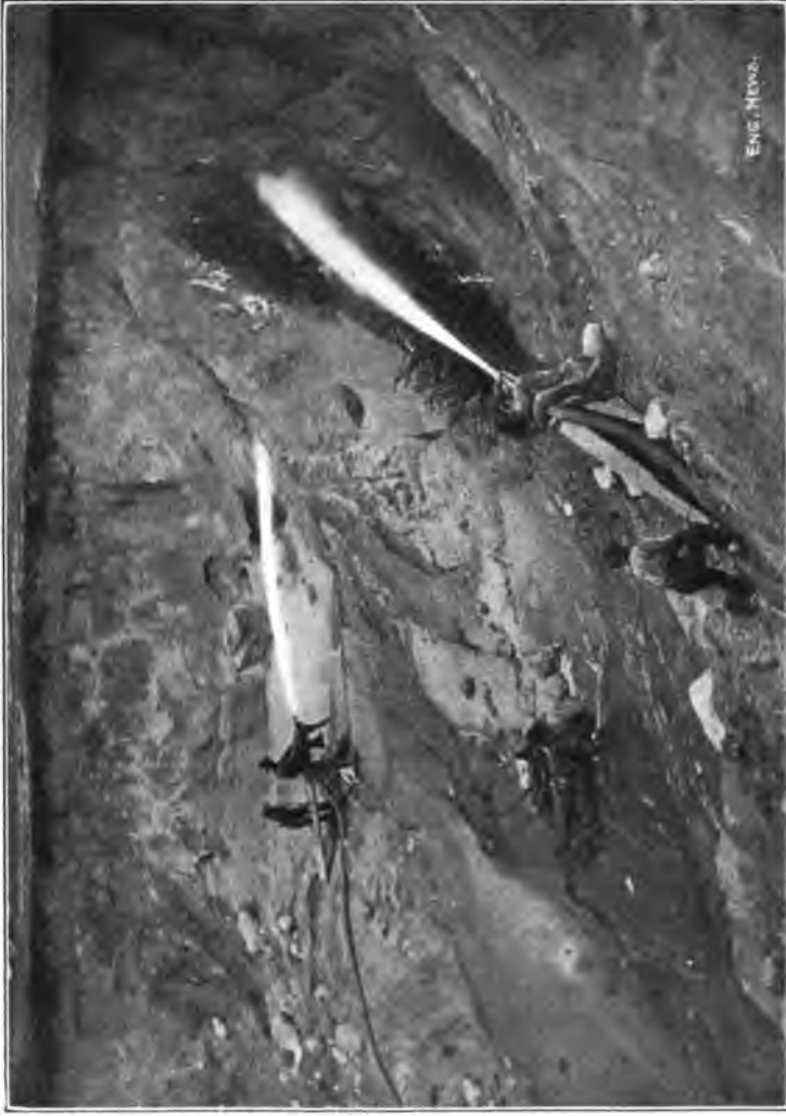
FIG. 139.—HYDRAULIC SLUICING ON THE CROTON DAM, SHOWING THE IMPROVED NOZZLE CONTROL, OR HYDRAULIC MONITOR. 181
