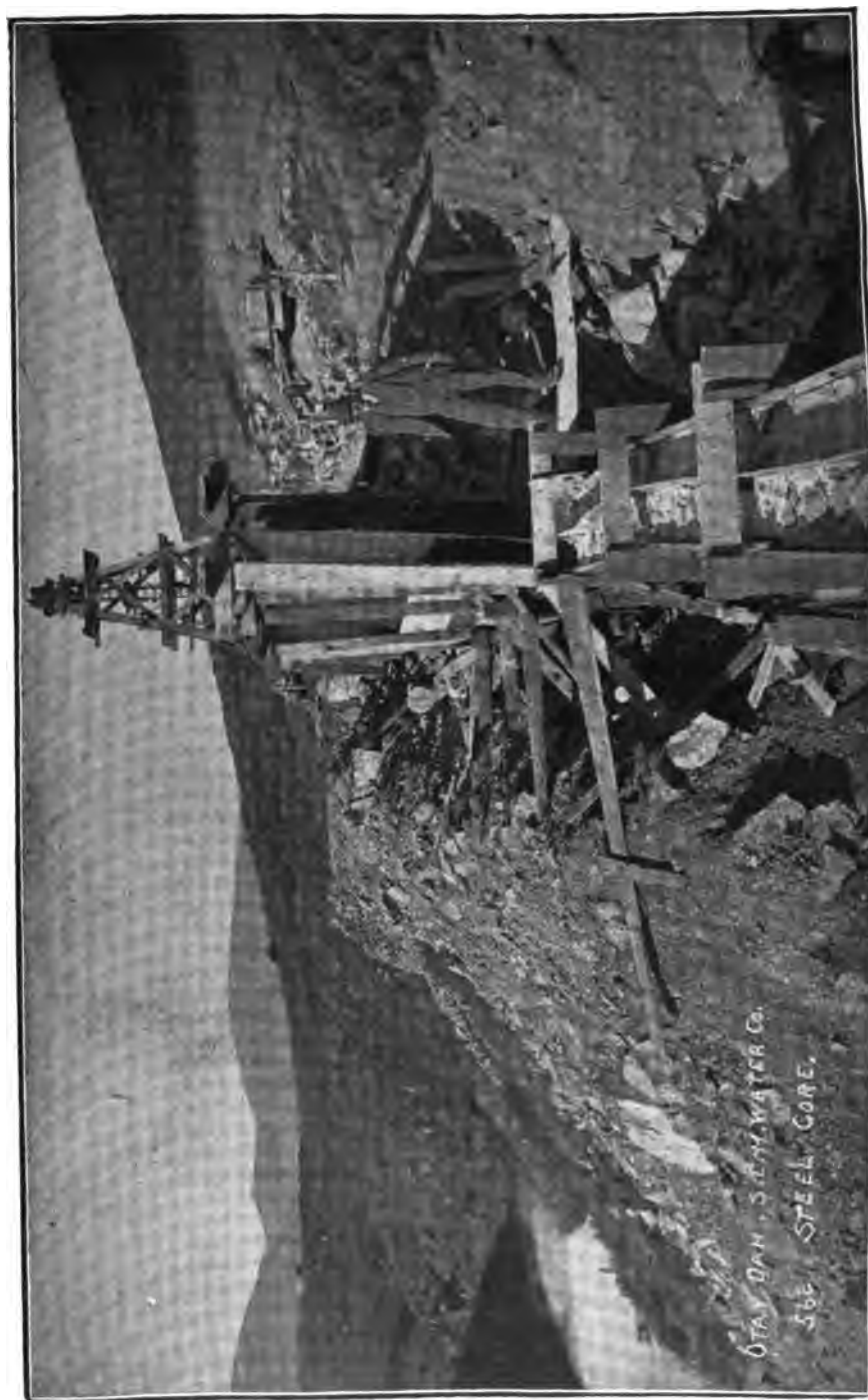
FIG. 15.—OTAY (CAL.) ROCK-FILL DAM -STEEL CORE.
