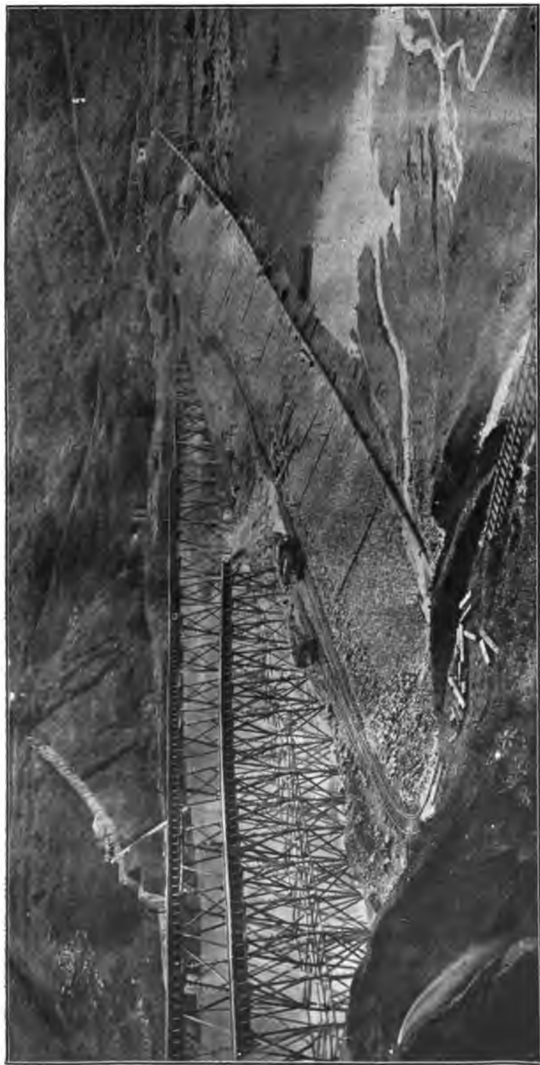
FIG. 128.—NECAXA DAM, MEXICO, OCT. 26, 1907, SHOWING MATERIAL BEING DEPOSITED BY FLUME. ALSO HYDRAULIC ELEVATOR OPERATING UNDER 700 FEET HEAD, LIFTING WATER FROM POND INTO POWER CANAL AT HEADWORKS AT END OF PIPE.
