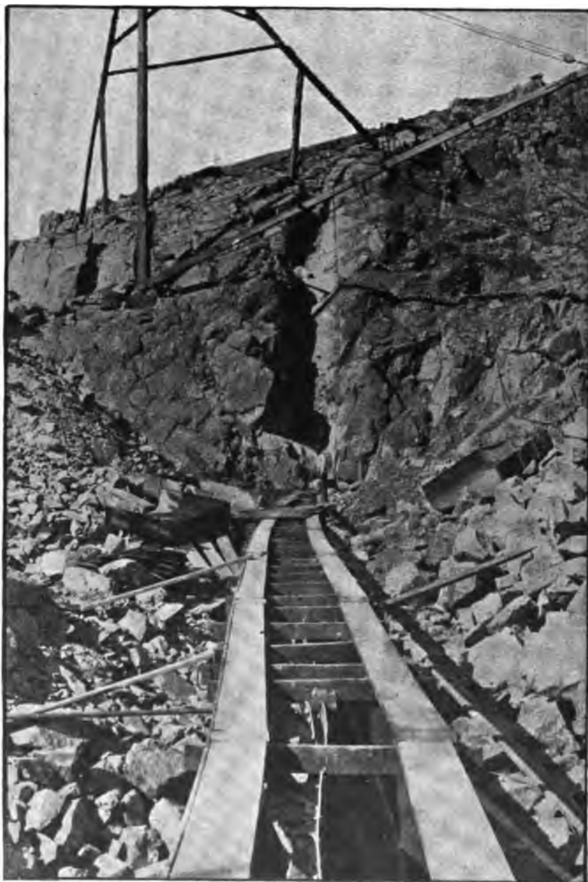
FIG. 14.—STEEL WEB-PLATE AND ANCHOR-TRENCH AT WEST END OF LOWER OTAY DAM.
