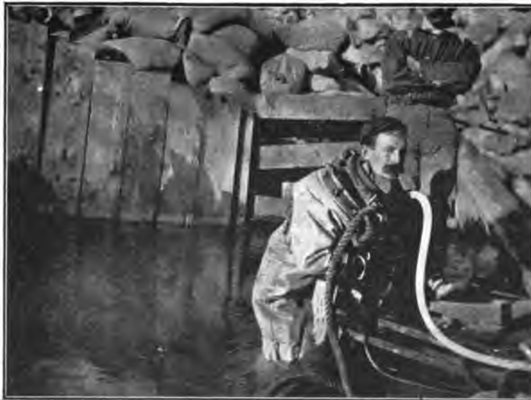
FIG. 50.—MILNER DAM. DIVERS AT WORK PLACING SHEET PILING IN 40 FEET OF WATER.
