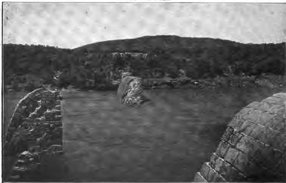
F.G. 231.—AUSTIN DAM, TEXAS, AFTER SUBSIDENCE OF FLOOD OF APRIL 7, 1900. Showing section of masonry moved bodily down-stream.
