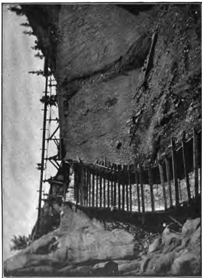
FIG. 106.—WASTEWAY FLUME FOR FLOOD DISCHARGE OVER LOWER SLOPE OF TERRACE DAM. SUMMER OF 1907.
