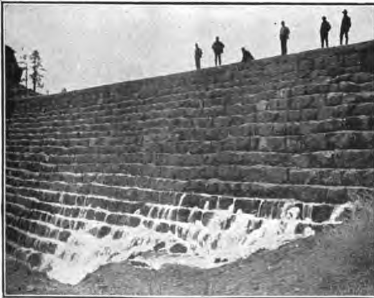
FIG. 30.—CASTLEWOOD DAM, COLO., SHOWING LEAKAGE THROUGH ROCK-FILL.
