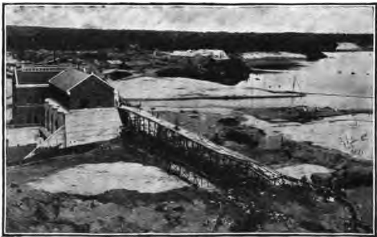
FIG. 137.—CROTON HYDRAULIC-FILL DAM, MICHIGAN, DURING CONSTRUCTION.
