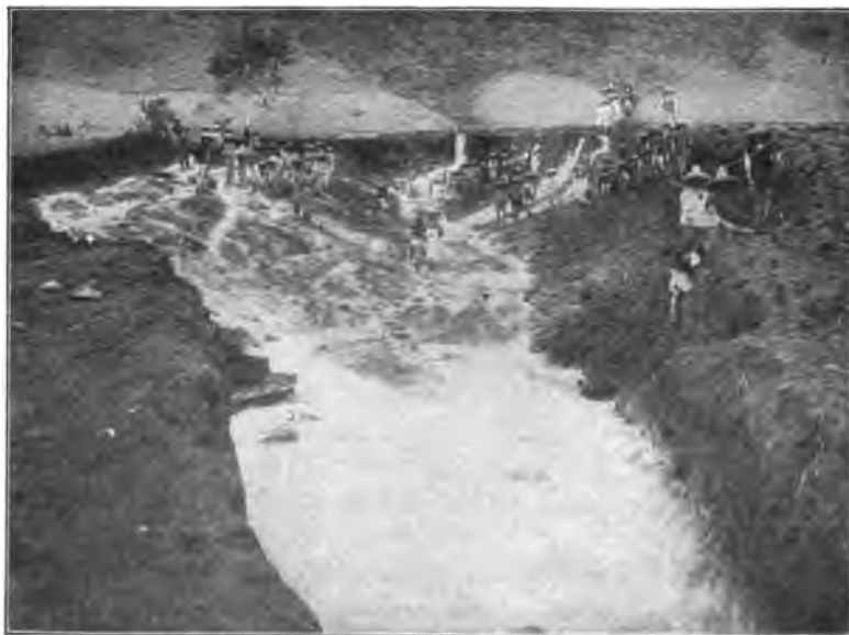
FIG. 131.—GROUND-SLUCING ON DAM NO. 1, TENANGO RIVER.
