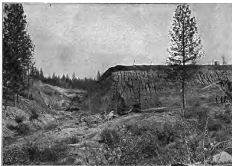
FIG. 84.—BREAK IN ORIGINAL LAKE FRANCES DAM. LOOKING UP STREAM.
