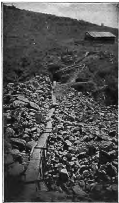
FIG. 16.—CREST OF LOWER OTAY DAM, SHOWING WEB-PLATE OF STEEL EMBEDDED IN CONCRETE. DAM NEARING COMPLETION.
