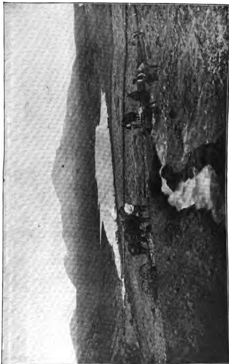
FIG. 71.—LA MESA (CAL.) DAM IN COURSE OF CONSTRUCTION BY THE HYDRAULIC PROCESS. Showing method of loosening earth to get it in suspension before taking it into carrying conduit. The conduit was built in 20-foot sections, which could be and were frequently taken apart and moved as conditions required.
