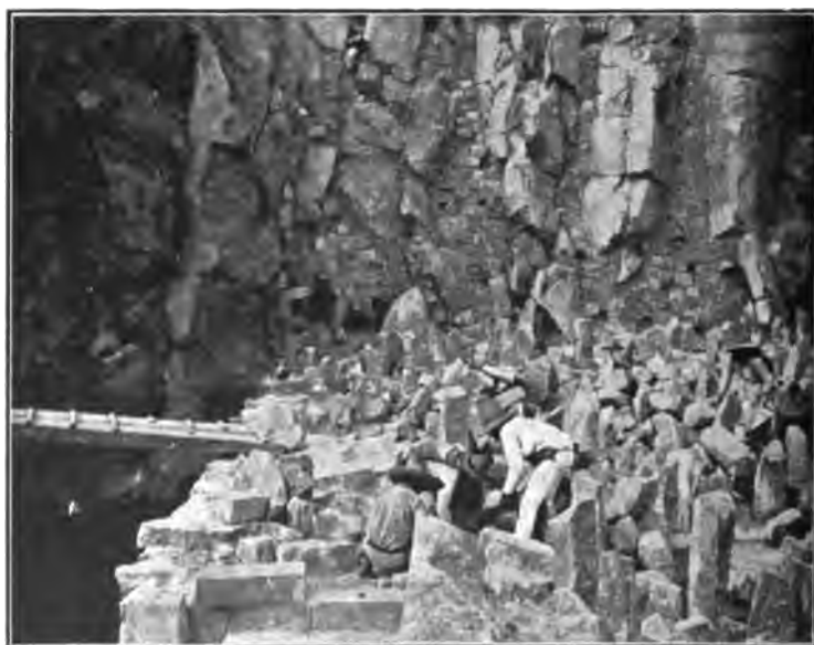
FIG. 375.—ILLUSTRATING THE BONDING OF THE MASONRY OF THE SAN JOSÉ DAM MEXICO.
