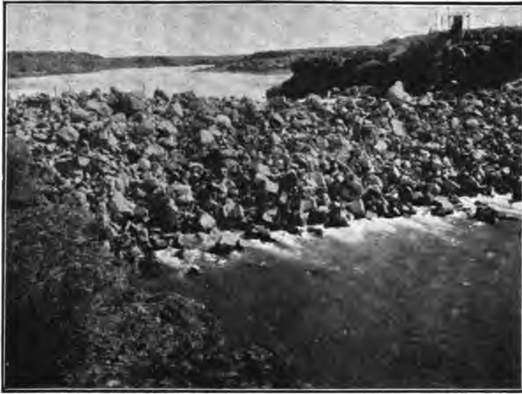
FIG. 49.—MILNER DAM, SNAKE RIVER, IDAHO. NORTH CHANNEL DAM BEFORE COMPLETION OF SHEET PILING. ABOUT 500 SECOND-FeET IS PASSING THROUGH ROCK-FILL, UNDER HEAD OF 13 FEET.
