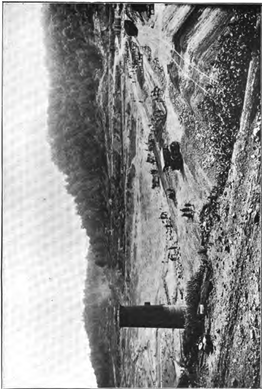
FIG. 359.—ILLUSTRATING THE STEEL OUTLET TOWER AND METHODS OF CONSTRUCTION OF THE HINKSTON RUN CINDER-FILL DAM, JOHNSTOWN, PA.
