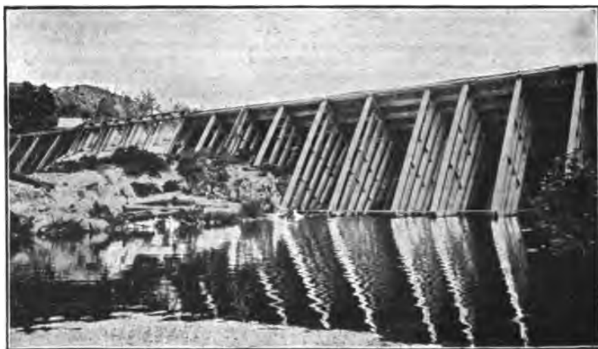
FIG. 342.—THE TIMBER WORK OF THE FAUCHERIE DAM AS SEEN FROM BELOW.
