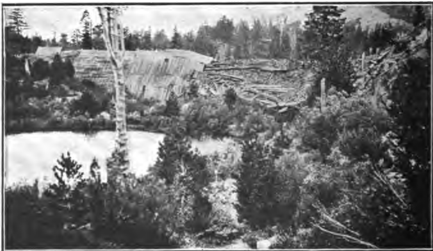
FIG. 347.—GENERAL VIEW OF THE TIMBER SKIN ON UP-STREAM SIDE OF THE ENGLISH LAKE DAM. NOW IN RUIN.
