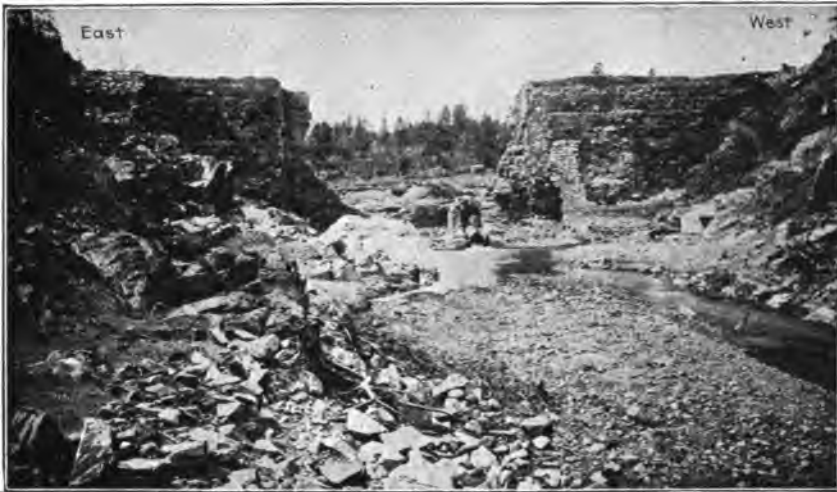
FIG. 209.—LYNX CREEK DAM, ARIZONA, AFTER RUPTURE BY FLOOD. VIEW FROM BELOW.
