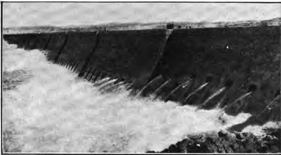
FIG. 267.—THE ASSOUAN DAM, EGYPT. SHOWING DISCHARGE THROUGH A NUMBER OF SLUICES.
