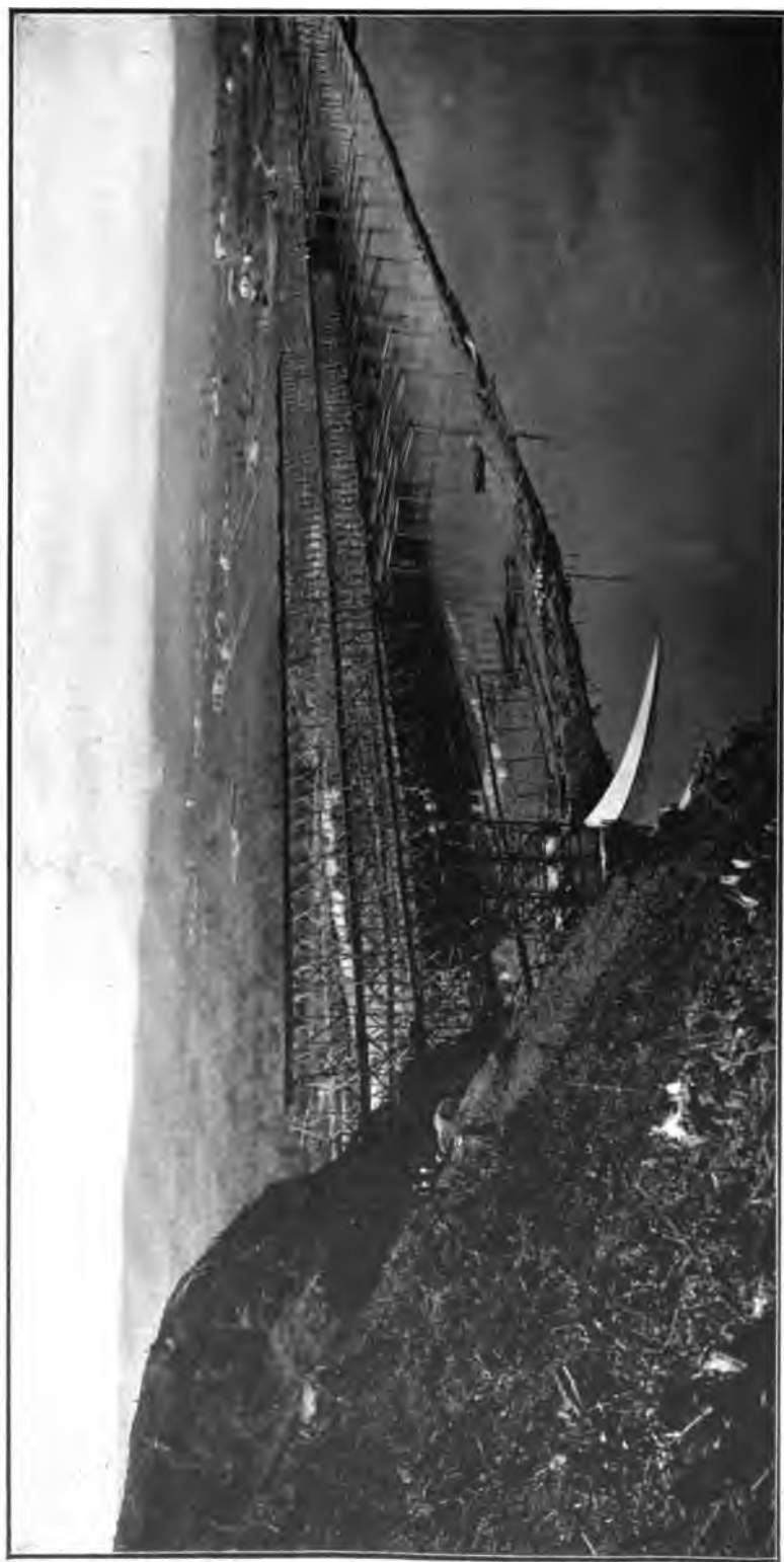
FIG. 109.—GENERAL VIEW OF SANTO AMARO DAM, BRAZIL, AUG. 21, 1907. SHOWING THREE LEVELS OF DELIVERY ON CENTRAL TRESTLE. TOTAL LENGTH 5300 FEET, MAXIMUM HEIGHT 63 FEET. 148
