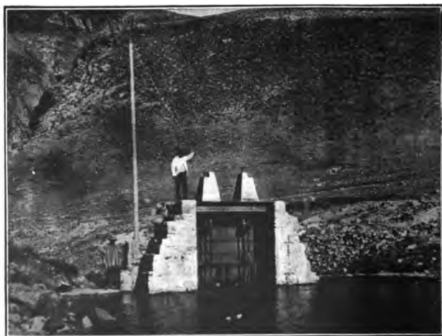
FIG. 279.—SACSA DAM, PERU, DESIGNED TO BE INCREASED IN HEIGHT 8 FEET, SHOWING GATES. 412
