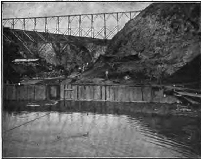
FIG. 99.—WAIALUA DAM, HAWAII. LOOKING DOWN-STREAM THROUGH DAM-SITE, SHOWING DIVERTING DAM AT UPPER TOE, AND TRESTLE FOR MAKING THE ROCK-FILL.
