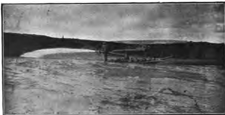
FIG. 60.—ZUÑI DAM, NEW MEXICO, SHOWING HYDRAULIC MONITOR IN ACTION.
