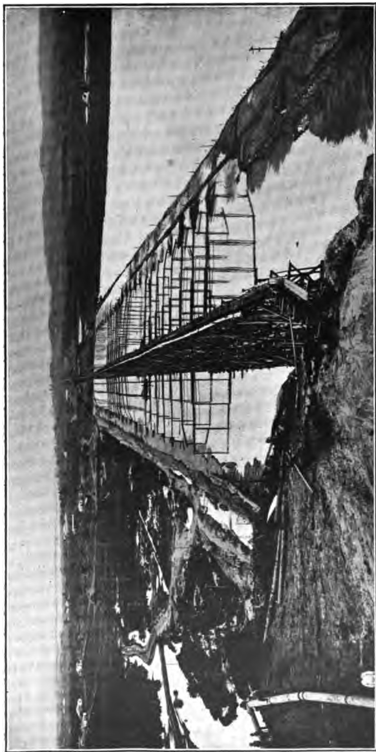
FIG. 108.—SANTO AMARO DAM, SAO PAULO, BRAZIL. (1 MILE LONG.) SHOWING METHOD OF DELIVERY OF SLUICED MATERIAL THROUGH FLUMES AND LATERALS.
