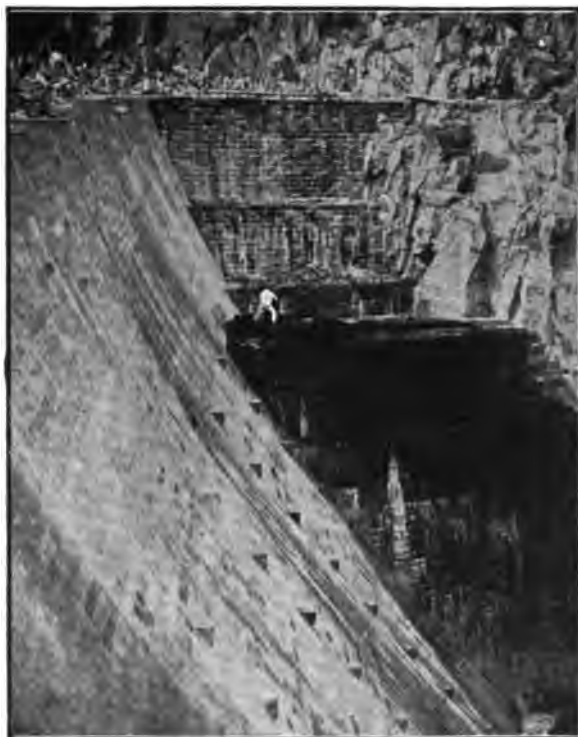
FIG. 373.—LOOKING ALONG THE FACE OF THE SAN JOSÉ DAM, AT SAN LUIS POTOSÍ, SHOWING FACE OF WALL SUPPORTING SIDE OF PRINCIPAL SPILLWAY.
