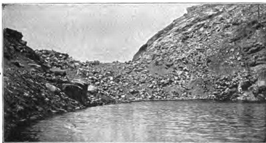
FIG. 22.—MORENA ROCK-FILL DAM IN PROCESS OF CONSTRUCTION. SHOWING TOP OF TOE-WALL ABOVE THE WATER-LINE.
