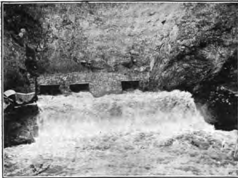
FIG. 97.—WAIALUA DAM, HAWAII, SHOWING FLOOD DISCHARGE THROUGH OUTLET TUNNELS DURING CONSTRUCTION, UNDER HEAD OF 8 FEET AT UPPER END OF TUNNELS.
