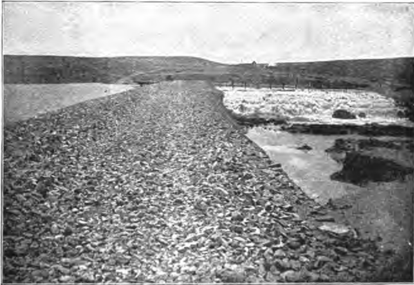
FIG. 34.—LAKE AVALON DAM, PECOS RIVER, NEW MEXICO SHOWING THE CREST OF COMPLETED DAM AND SPILLWAY DISCHARGING.
