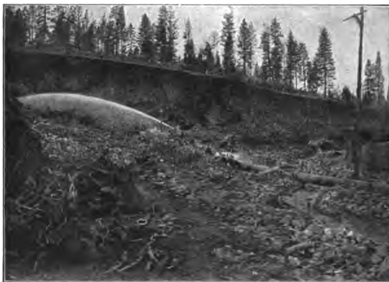
FIG. 89.—HYDRAULIC GIANT IN ACTION UNDERCUTTING THE BANK.
