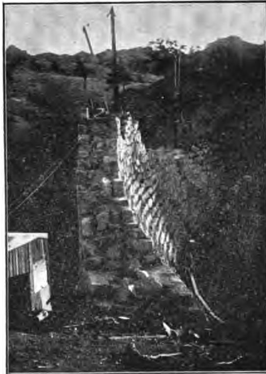
FIG. 233.—GRANITE SPRINGS DAM, WYOMING. SHOWING GENERAL CHARACTER OF RUBBLE MASONRY.
