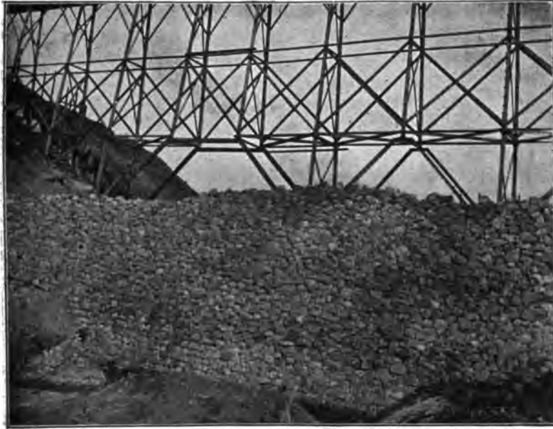
FIG. 96.—ROCK-FILL ON DOWN-STREAM SIDE OF WAIALUA DAM.
