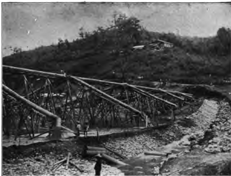
FIG. 130.—LIQUID EARTH BEING DEPOSITED THROUGH PIPES ON OUTER SLOPES OF DAM NO. 1, TENANGO RIVER.
