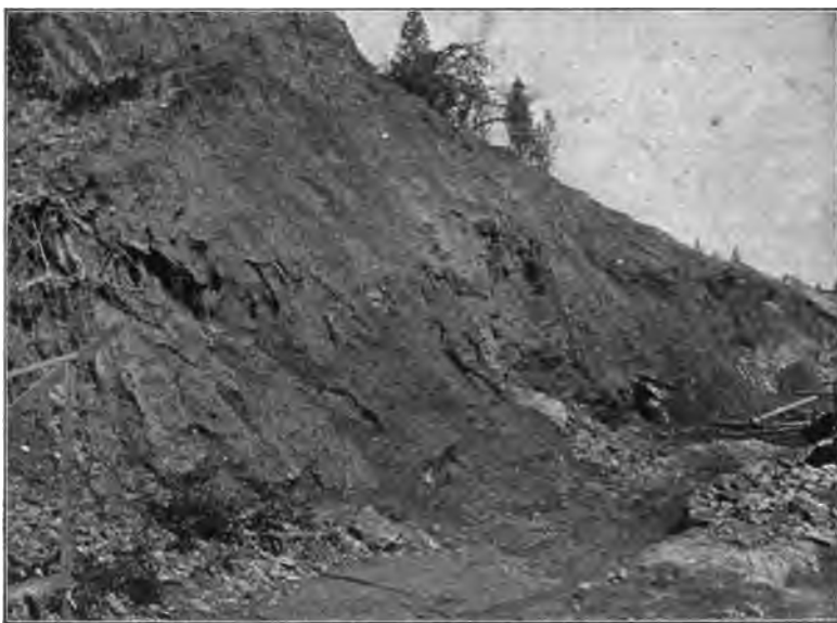
FIG. 85.—NEAR VIEW OF RIGHT SIDE OF BREAK IN EMBANKMENT OF LAKE FRANCES DAM SHOWING ROOTS EXPOSED BY THE BREAK.
