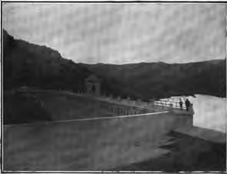
FIG. 258.—MERCEDES DAM, MEXICO, LOOKING ACROSS SPILLWAY CHANNEL, SHOWING CURVED PORTION AT FAR END.
