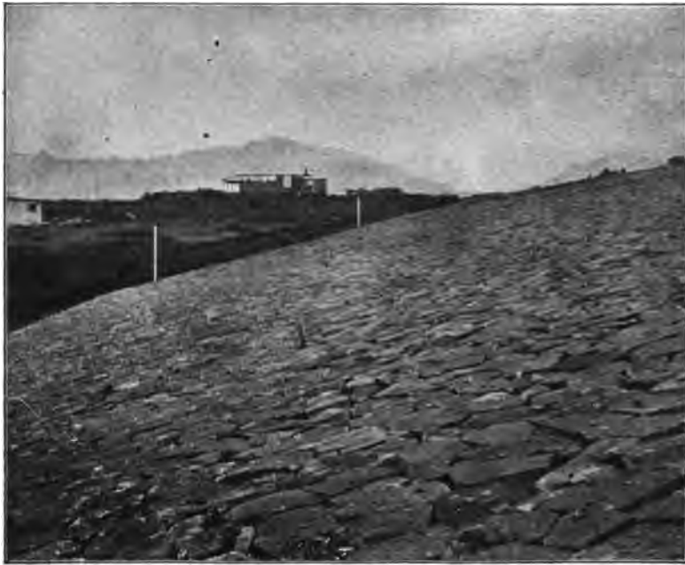
FIG. 98.—RIP-RAP ON FACE OF HYDRAULIC-FILL, WAIALUA DAM.
