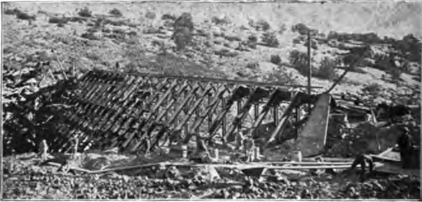
FIG. 295.—ASH FORK, STEEL DAM, SHOWING FRAME READY TO RECEIVE PLATES.
