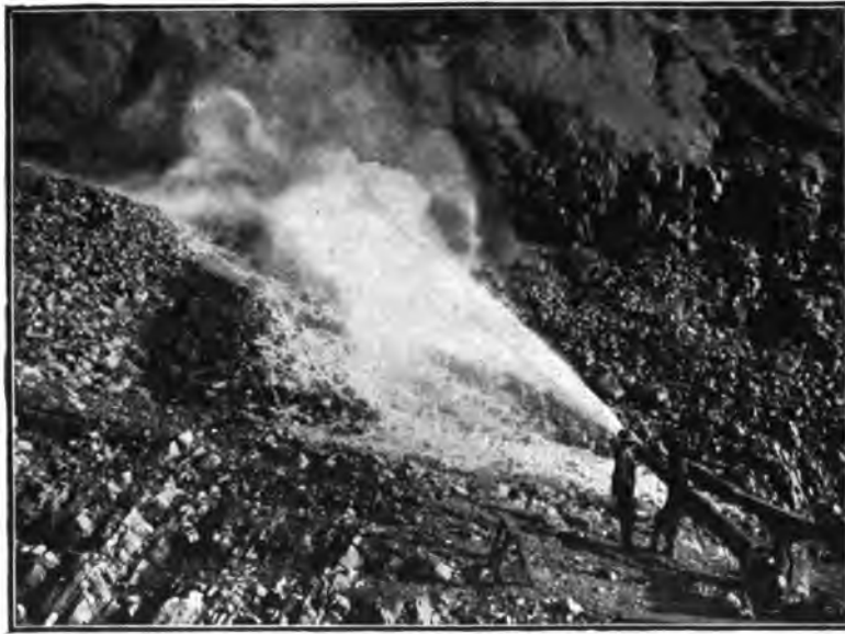
FIG. 117.—HYDRAULIC MONITOR WORKING ON LINE OF CONTACT BETWEEN LIMESTONE AND LAVA IN SPILLWAY CUT, NECAXA DAM, MEXICO.
