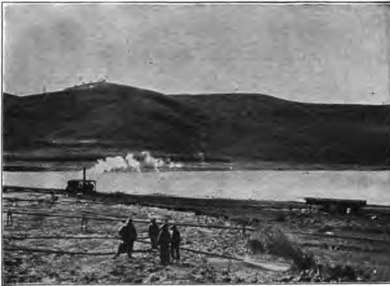
FIG. 136.—SILVER LAKE DAM, LOS ANGELES. THE EARTH, LOOSENED BY THE HYDRAULIC JET, IS CONVEYED TO THE PUMPING STATION SHOWN AND PUMPED TO THE DAM.
