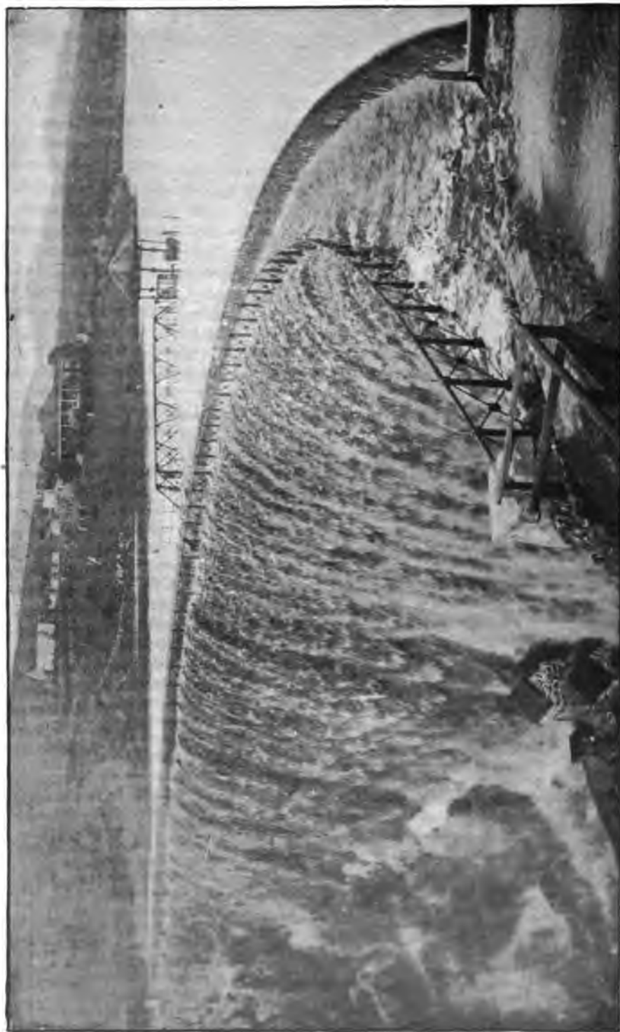
FIG. 155.—SWEETWATER DAM DURING THE GREAT FLOOD OF JANUARY 17, 1895.
