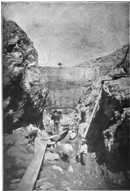
FIG. 11 — MASONRY FOUNDATION OF LOWER OTAY DAM.
