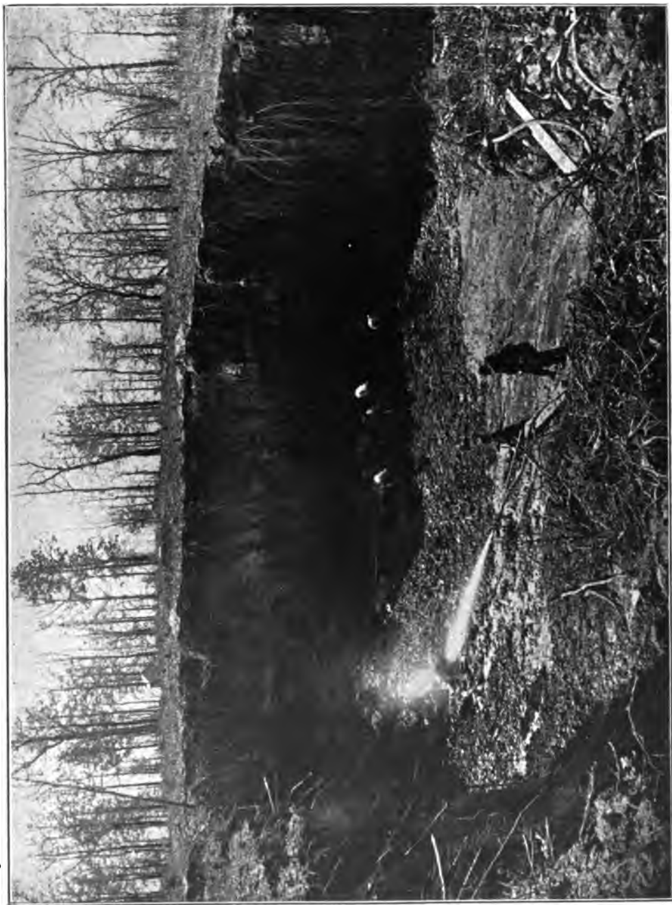
FIG. 68.—HYDRAULIC SLUICING FOR BUILDING DAM AT TYLER, TEXAS.
