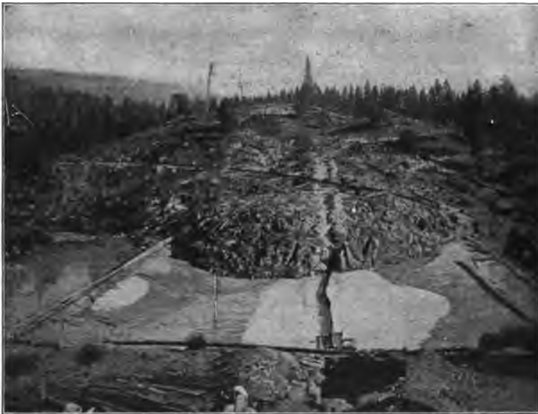
FIG. 79.—CRANE VALLEY DAM. SHOWING WOODEN FENCE, OR CENTER DIAPHRAGM, WHICH WAS CARRIED UP TO A HEIGHT OF 30 FEET ABOVE BED-ROCK.
