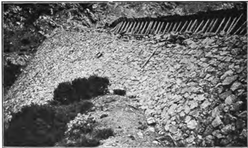
FIG. 348.—THE DOWN-STREAM FACING OF THE ENGLISH LAKE DAM, CONSISTING OF A HAND-LAID DRY WALL IS WELL ILLUSTRATED BY THIS PHOTOGRAPH.
