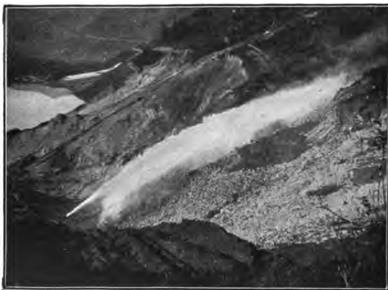
FIG. 115.—NECAXA DAM, MEXICO. HYDRAULIC MONITOR WORKING UNDER 180 POUNDS PRESSURE, 6-INCH NOZZLE, 30 SECOND-FEET OF WATER.
