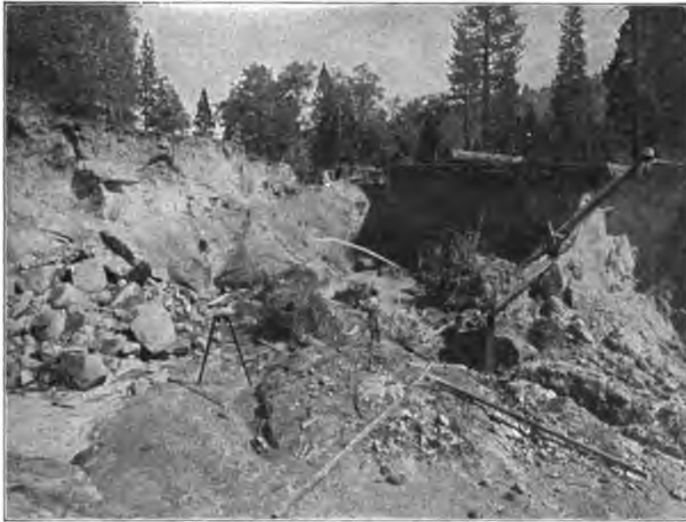
FIG. 81.—CRANE VALLEY HYDRAULIC-FILL DAM. SHOWING METHOD OF LOOSENING THE MATERIALS SLUICED INTO THE DAM.
