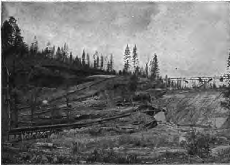
FIG. 88.—WEST END OF LAKE FRANCES DAM, SHOWING THE BREAK RESTORED, THE HIGHER DAM NEARLY COMPLETED, THE HYDRAULIC GIANT AT WORK, AND THE MAIN PIPE LINE SUPPLYING WATER TO THE PUMP.
