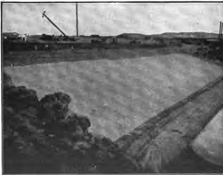
FIG. 56.—HYDRAULIC-FILL SIDE OF ZUÑI DAM. SHOWING GRAVEL COVER OF STONE RIPRAP.
