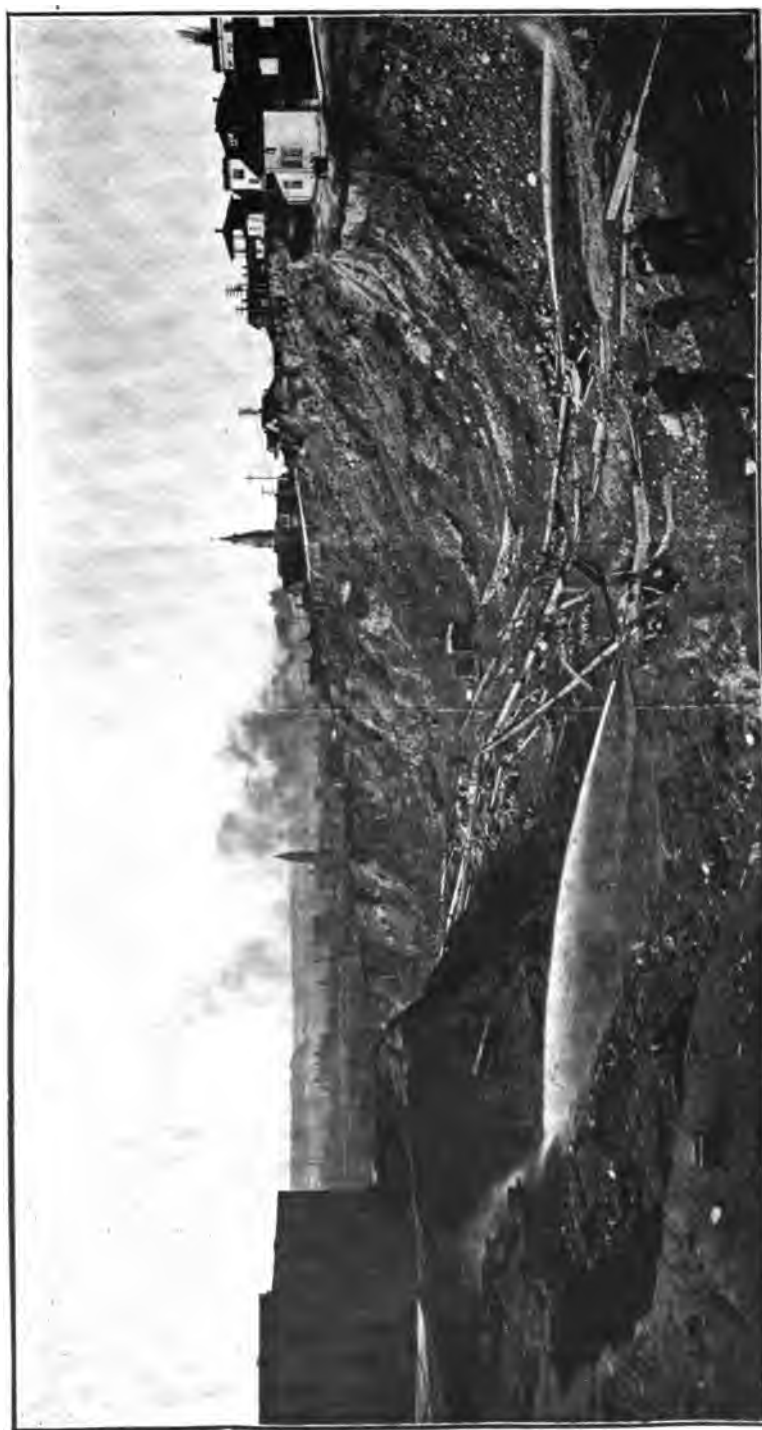
FIG. 353.—THE JACKSON STREET REGRADE BY HYDRAULIC SLUICING, WITH WATER PUMPED.
