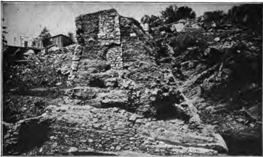
FIG. 210 —LYNX CREEK DAM, ARIZONA. SECTION SHOWING FACING WALLS AND CONCRETE HEARTING.
