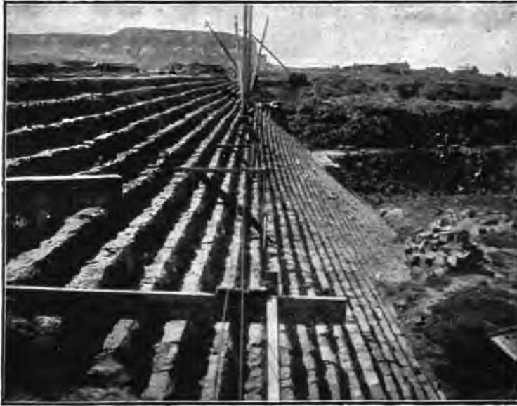
FIG. 55.—DOWN-STREAM FACE OF ZUÑI DAM. SHOWING CHARACTER OF DRY MASONRY IN THE ROCK-FILL.
