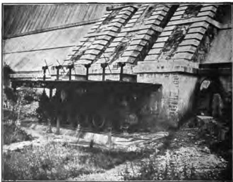
FIG. 366. —THE SIX OUTLET PIPES AND GATE-VALVES OF THE ESPERANZA DAM, BEFORE CONNECTION WITH WATER MAINS OF CITY.
