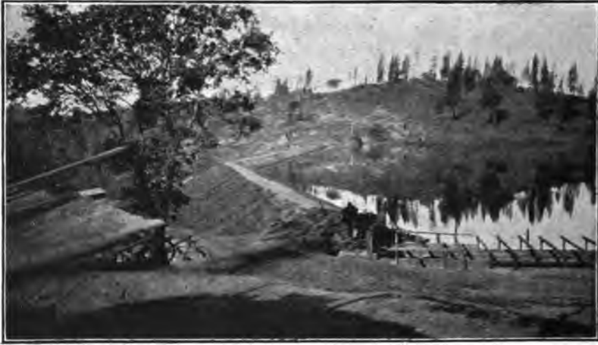
FIG. 349.—THE LAKE FRANCES HYDRAULIC-FILL DAM AS COMPLETED AND IN SERVICE, SHOWING NEW SPILLWAY AND GATES IN FOREGROUND.
